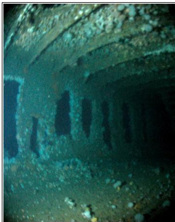
Figure 1-1: Deterioration of hull plating inside the Norness (Image: Sea Turtle Charters Facebook page).
