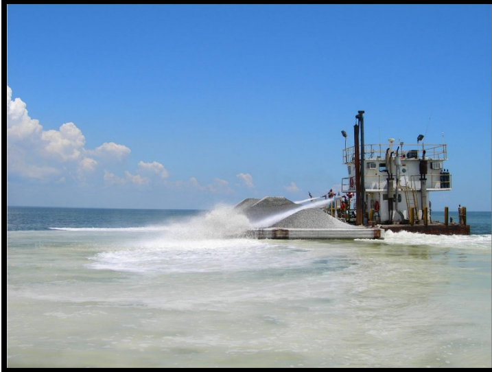
A barge of limestone being deployed by MSDMR to create an inshore reef. Photo Credit: GSMFC.
