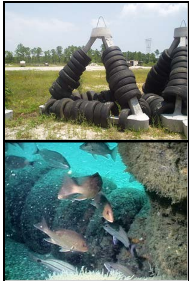
Concrete and tire tetrahedron modules that were deployed offshore Alabama from the mid-1990s-2010s. Photo Credit: ADCNR
