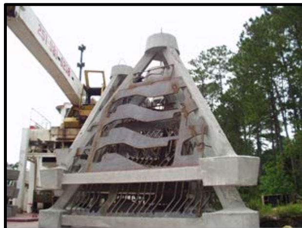
Concrete tetrahedron modules that incorporated steel cutouts from manufacturing operations were deployed offshore of Alabama and Florida from the mid-1990s-2010s. Photo Credit: ADCNR
